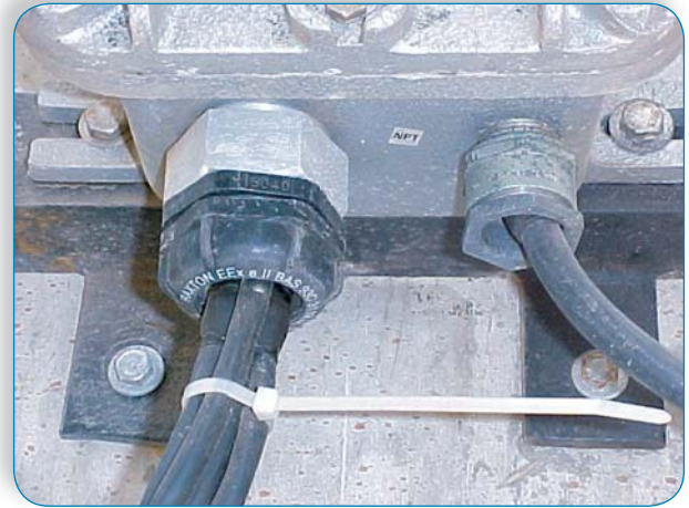
Fig. 2: The cable glands.
